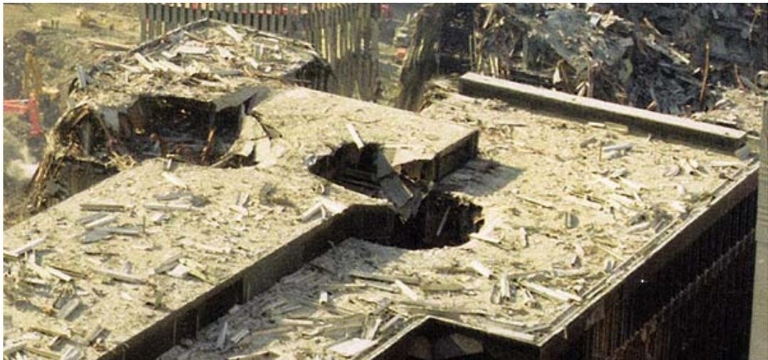
This further enlargement, the un-scarred roof segments overhanging the holes (arrows) suggest that the collapse originated from within:
