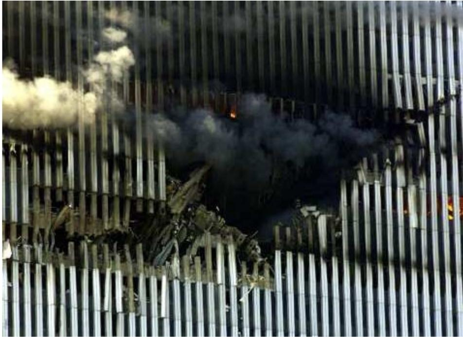
This photograph, like [others showing the towers' impact holes](#) does not show outward-bent steel columns, only outward-bent aluminum cladding.
