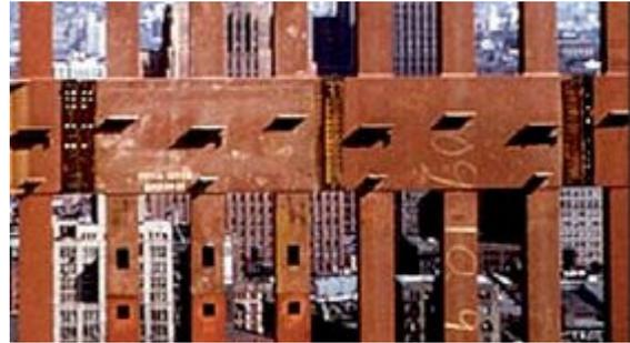
The upper photograph shows a row of floor trusses, and the lower photograph shows the steel shelves on which they rested. Eagar's description of these as "angle clips" is a gross misnomer.
